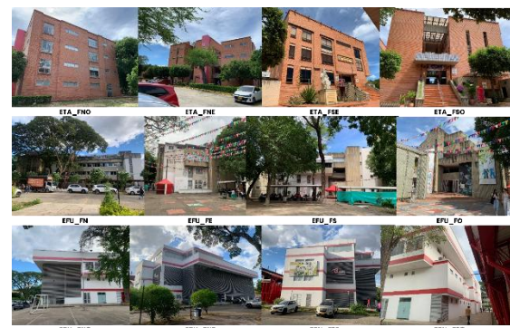
Fig. 3. Representative façades of the selected case studies after classifying the buildings according to the number of floors, main façade materials, and construction stage.
