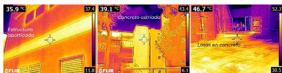
Fig. 5. Thermographic images of façade and surrounding surfaces: reinforced concrete frame structure (left), fluted concrete (center), concrete slab floors (right).
