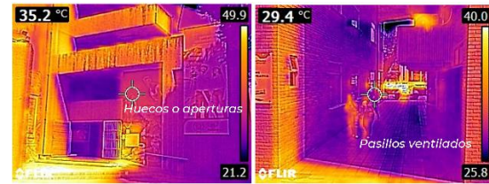
Fig. 6. Thermographic images of openings and naturally ventilated corridors in buildings.
