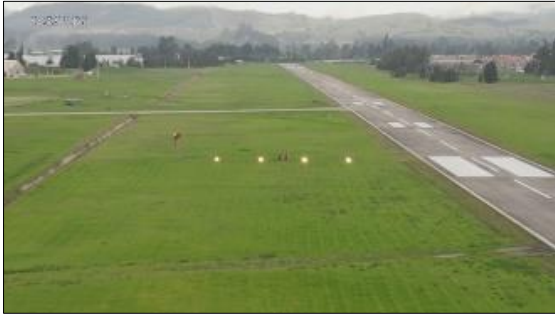
Fig. 1. PAPI lights setup Source: Own image
