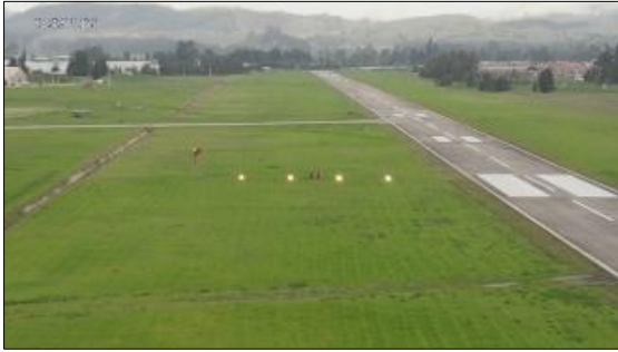
Fig. 1. PAPI lights setup Source: Own image
