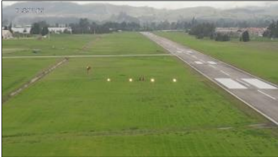
Fig. 1. PAPI lights setup Source: Own image
