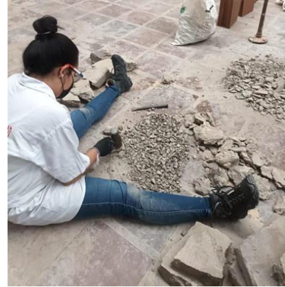
Fig. 2. Crushing RCD Manual. Source: own production.
