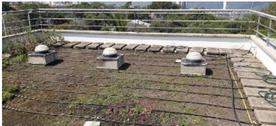
(a) Laying of the irrigation network.
