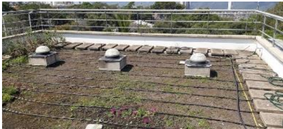
(a) Laying of the irrigation network.
