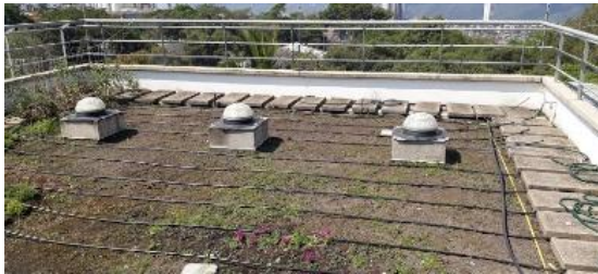
(a) Laying of the irrigation network.
